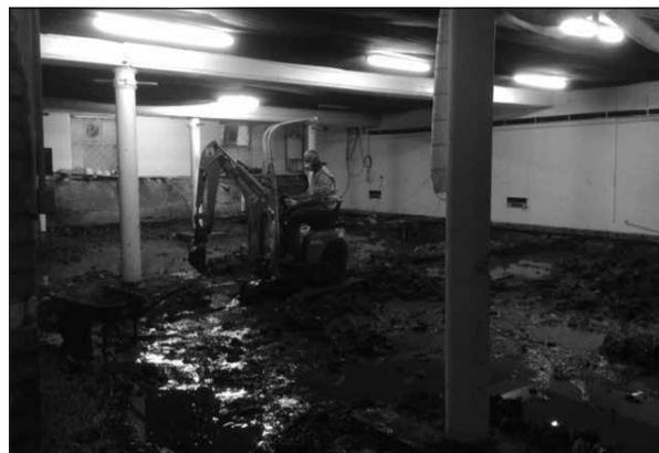
**Digging in:** Work in progress in early November on the basement floor, which is being lowered and waterproofed.
